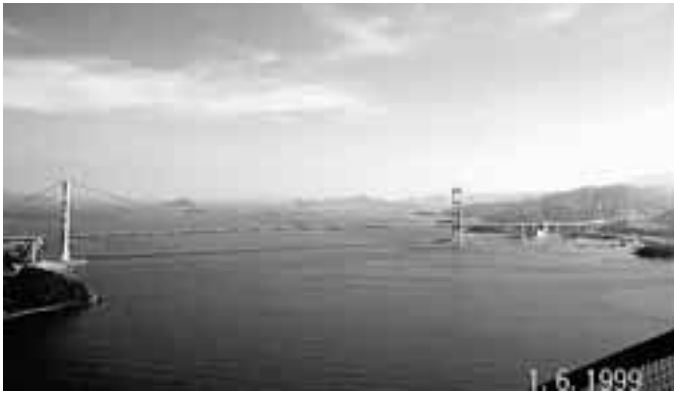
Fig. 10. Tsing Ma Bridge (Hong Kong)
